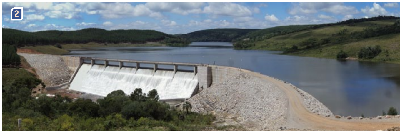
2. Barragem e represa | Dam and reservoir
